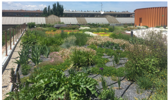
Figure 33. View of Europa Congress Centre's green roof.
