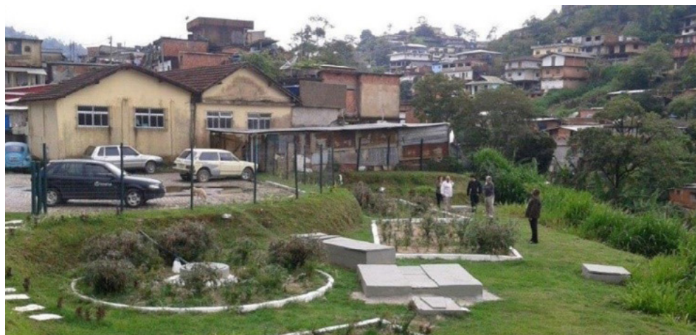
Figure 59. Nature-based solution to treat waste water: biogas digester and built wetland in Vila Ipanema, Petrópolis.
