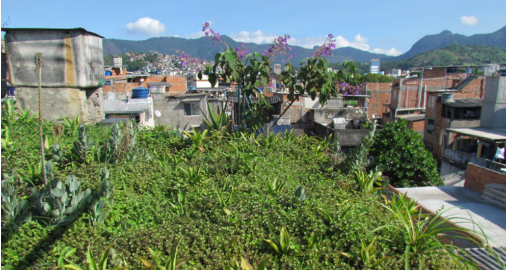
Figure 72. Green roof at the Arará community in the heart of a highly built-up and paved area with extremely hot temperatures all year round.
