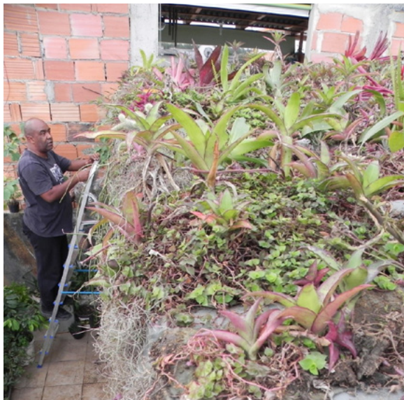
Figure 73: Detail of the green roof at the Arará community: native bromeliads are some of the chosen species.
