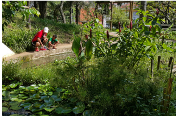
Figure 64. Built pond to collect the water from the eight springs of the Água Preta creek — social ecological benefits in the heart of the city.
