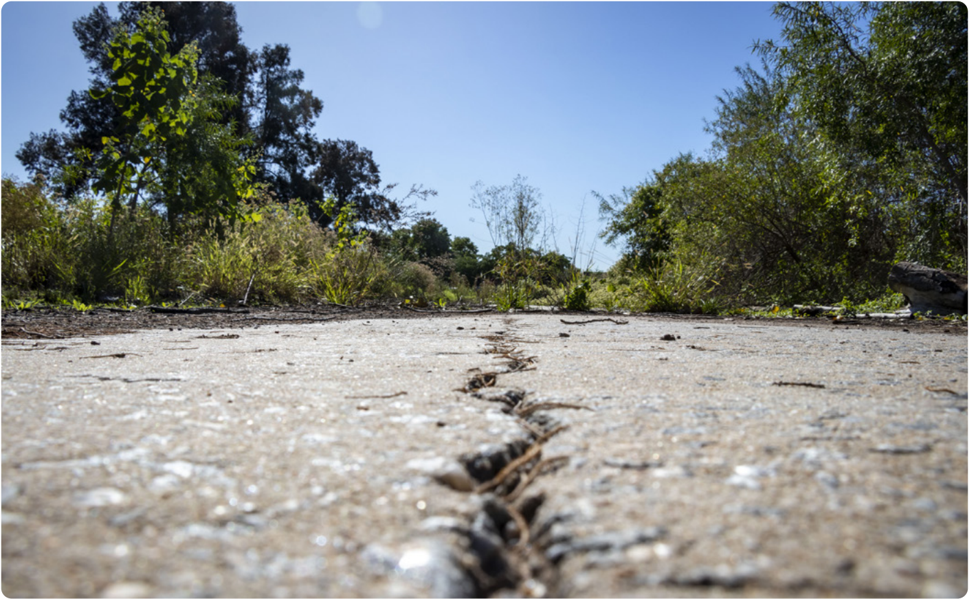
Remaining paving prior to the full wetland works. April 28, 2022
