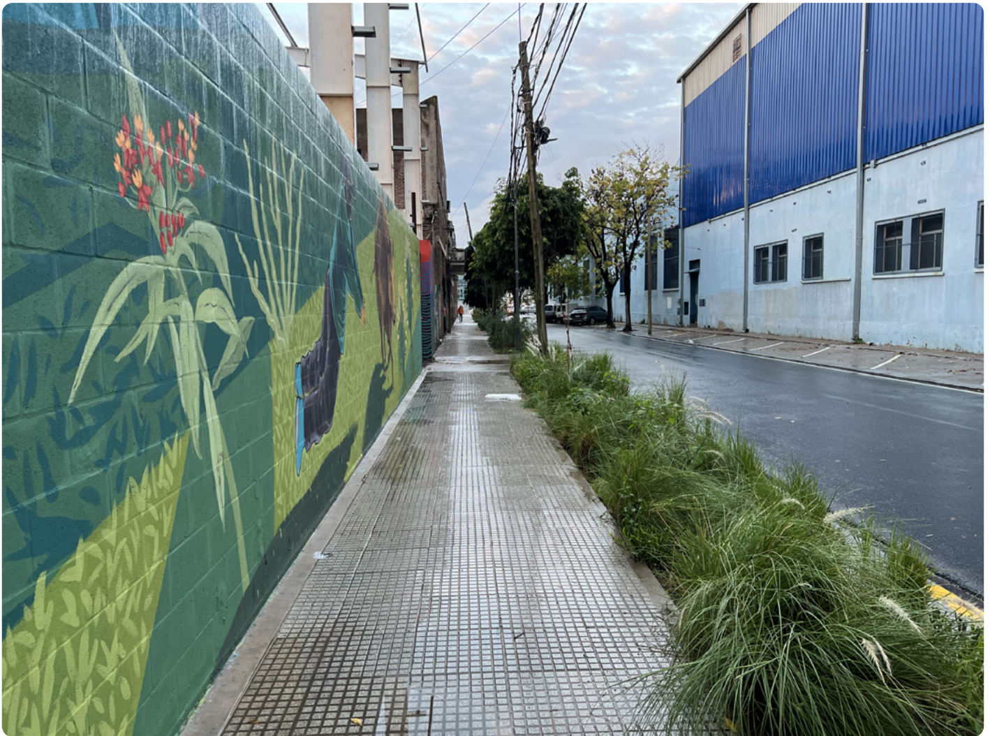
Rain gardens in the context of the comprehensive upgrading works along Francia Street
